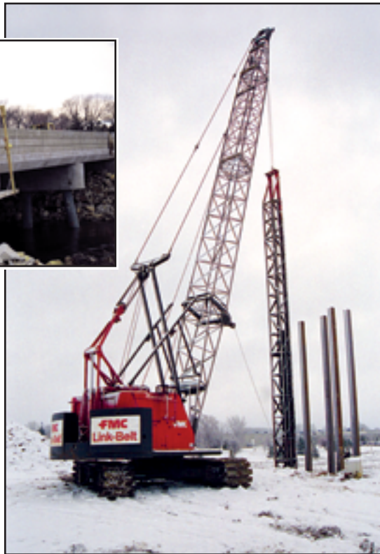
Using this Link-Belt crane, a Minnowa operator drives a pile at a bridge job near Highway 63 in New Hampton, Iowa.
