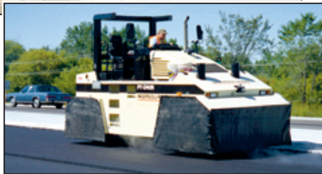
Crews working on a recent Superpave project on Highway 13 utilized a 25-ton Ingersoll-Rand PT240 rubber-tired roller.
