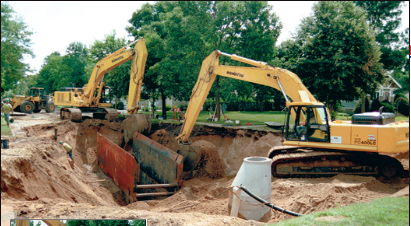
Above: Operators of Komatsu PC600LC-6 and PC400LC-6 excavators work in tandem to dig trenches on the River Falls utility project while the operator of a WA450-5 stockpiles material in the background. The large project included replacing sanitary sewer, storm sewer and water main lines in the city, as well as curb, gutter and street reconstruction work. Left: Foreman Marty Durdahl guided the work of crews at the River Falls job, the largest project to date for Three Rivers Construction.
