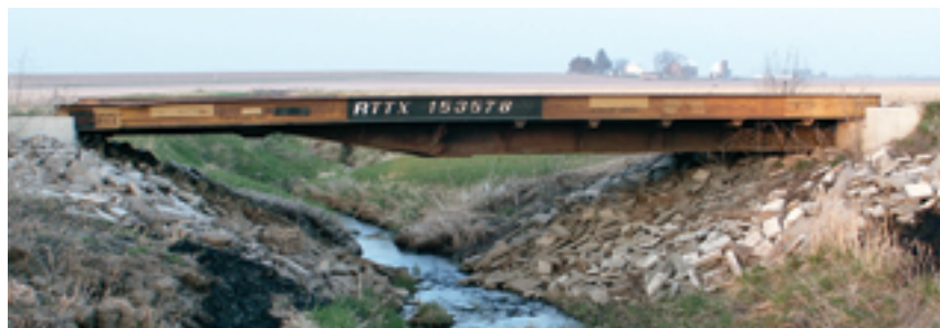
This bridge on a farm operation near Stanwood, Iowa, was constructed out of railroad cars. It's one of the unique agricultural improvement projects completed by Wynkoop Equipment Co.
