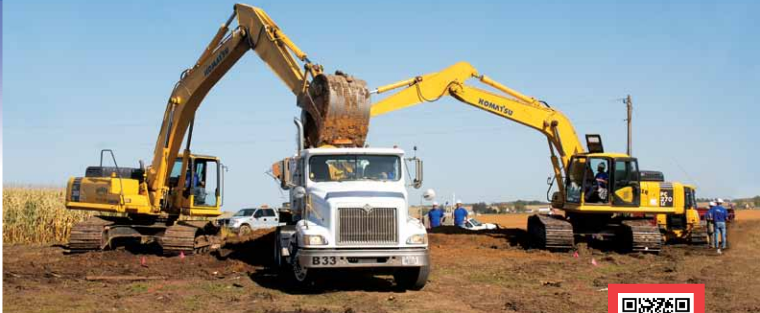
Working in tandem, Baker Concrete & Excavating operators use Komatsu PC300 and PC270 excavators to load dirt from the basement excavation for an Extreme Makeover home in West Union, Iowa. "Komatsu excavators have been our main production machines for many years because they're productive and reliable," said Owner Steve Baker.
