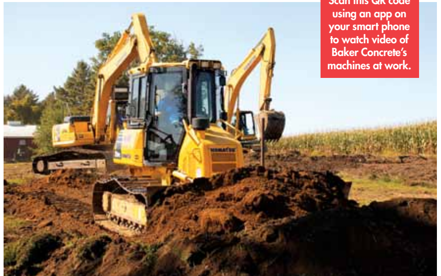
Working in tandem, Baker Concrete & Excavating operators use Komatsu PC300 and PC270 excavators to load dirt from the basement excavation for an Extreme Makeover home in West Union, Iowa. "Komatsu excavators have been our main production machines for many years because they're productive and reliable," said Owner Steve Baker.
