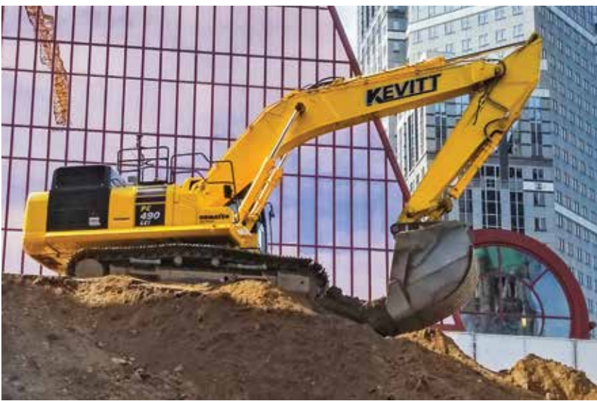
Using a Komatsu intelligent Machine Control PC490LCi-11, a Kevitt Excavating operator digs footings at the Minneapolis Public Services building.
