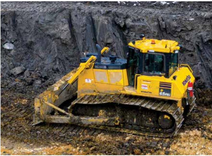
A Weber Stone Company operator uses a Komatsu D65PXi dozer with intelligent Machine Control to strip overburden and create a road.
