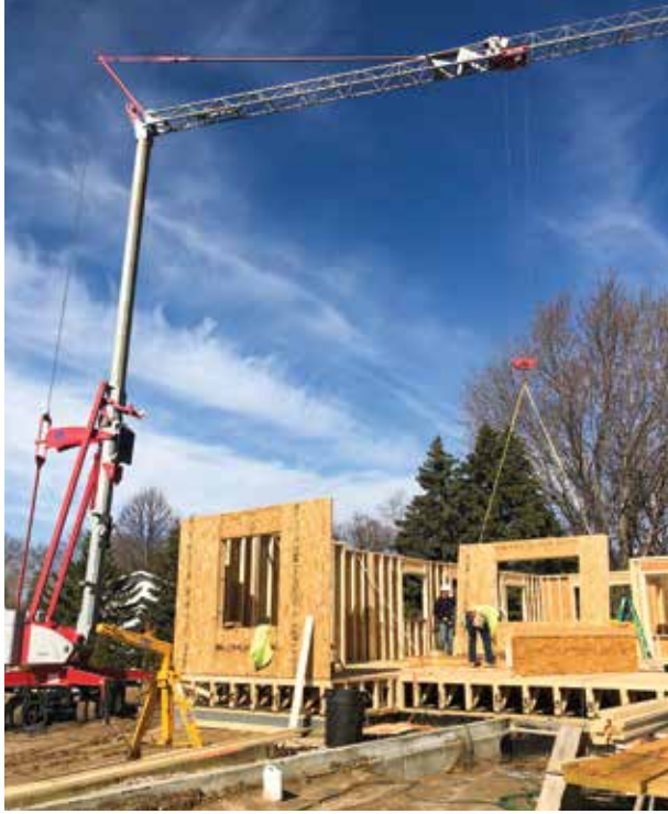
Link Construction, Inc., uses a Potain Igo MA 21 self-erecting crane from RMS Rentals to set a wall for a home in Shakopee, Minn.
