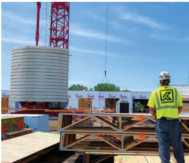
A Frana Companies, Inc. crane operator makes a supply drop remotely with a Potain Igo T 85 A self-erecting crane. "Our operators are busy all of the time," said Equipment Manager Kelly Anderson. "They can be anywhere on the site contributing to the work."
