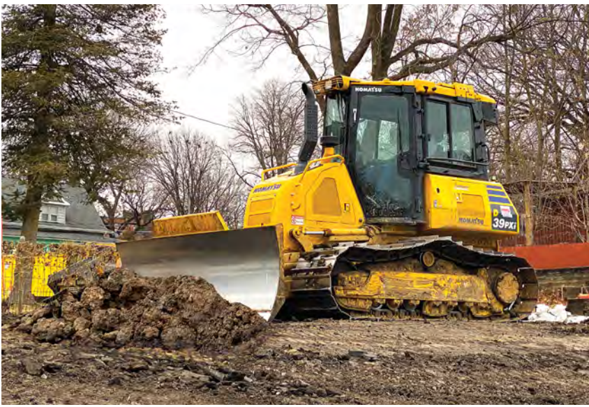
At a job site in Des Moines, a Synergy Contracting operator uses a Komatsu intelligent Machine Control D39PXi dozer to final grade.
