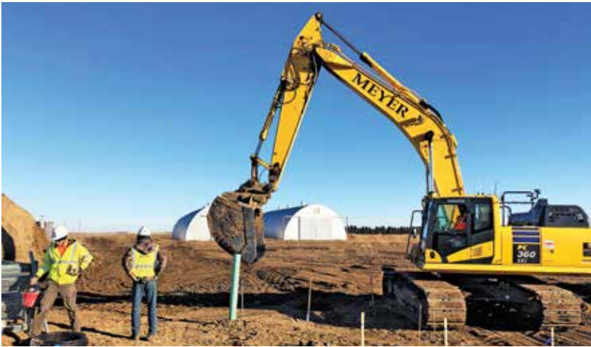
Meyer Contracting uses a Komatsu PC360LCi iMC excavator to work quickly and efficiently. "We can get to the bottom of the cut and dig footings much faster. We get exactly to grade, and we don't waste any material. Using iMC has been a huge savings for us operationally," said Vice President Mark Conte.
