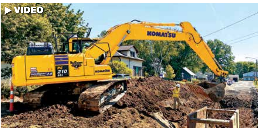
A DeCook Excavating crew places a trench box with a Komatsu PC210LCi-11 intelligent Machine Control (iMC) excavator on a street reconstruction project in Byron, Minn.
