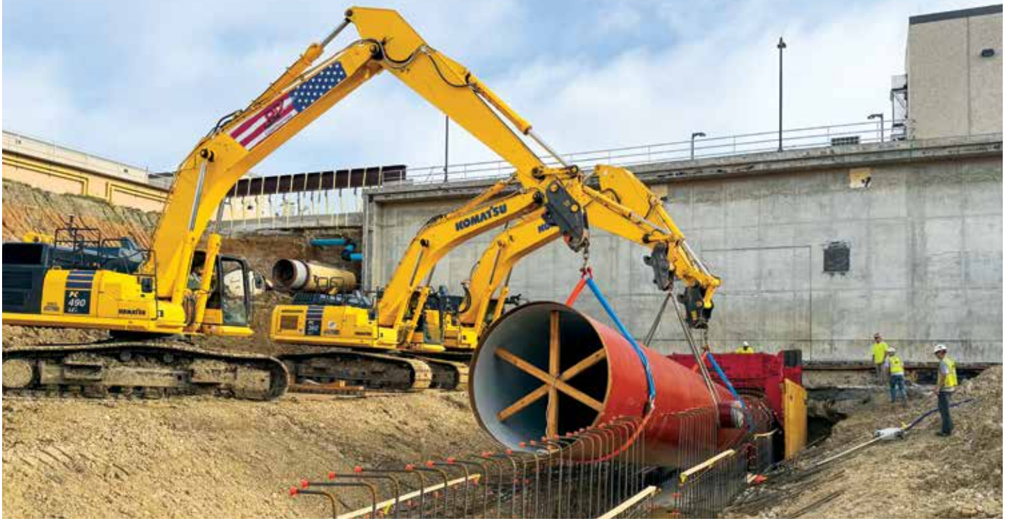
A trio of RP Constructors' Komatsu excavators work in tandem to place a section of pipe. Jobs like this are what RP Constructors seeks out. "The more complex it is, the better it is for us," said Vice President Travis Thom.
