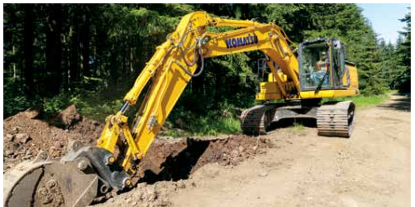
Komatsu's PC220LCi-12 intelligent machine control (IMC) 3.0 excavator now features swing-to-line and travel-along-line functions that help operators work more efficiently.
