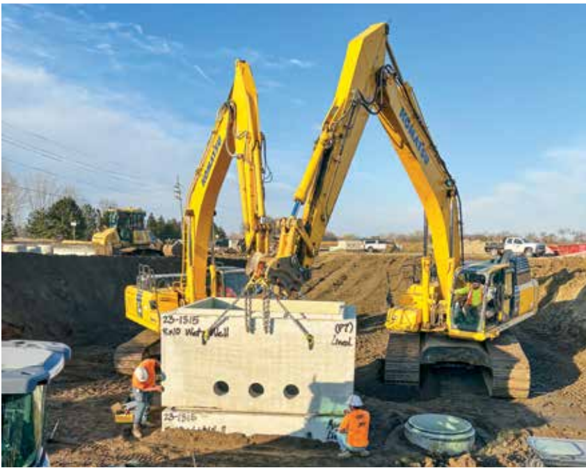
Using a pair of Komatsu excavators, RP Constructors lowers an 8-by-10-foot water well into place.
