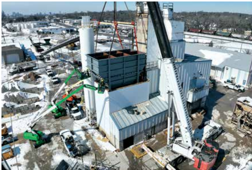
A recently completed project for Cemstone highlights RMS Tritec's ability to take on complex work and deliver with speed, precision and coordination.
